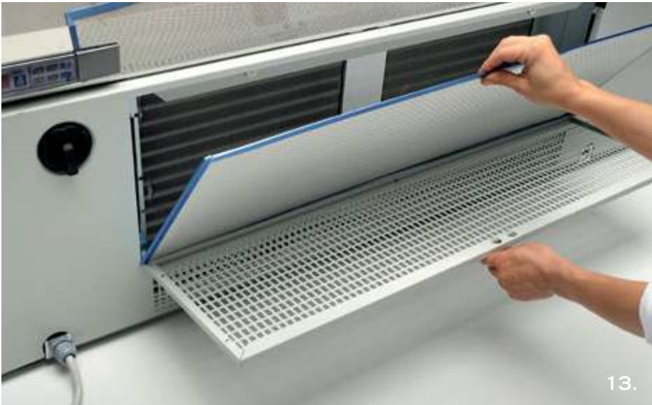
Condensing Unit Easy Cleaning
